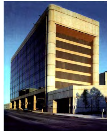
Fig. 1—Murrah Building Prior to Blast.
