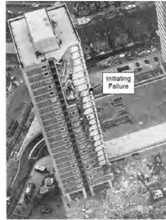
Figure 1-1 Ronan Point collapse: a gas explosion on the 18 th floor resulted in a progressive collapse
