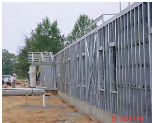
Load Bearing Wall Application
