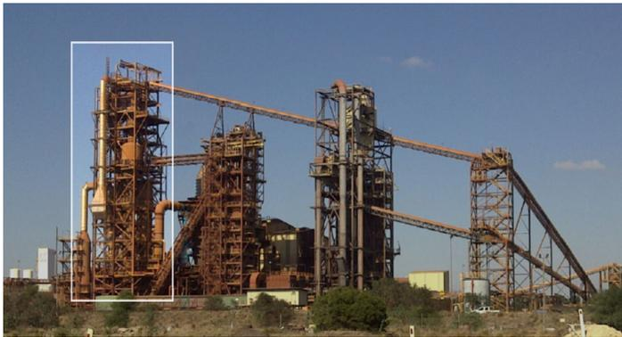
The nonlinear dynamic analysis performed by ASI in Extreme Loading® for Structures considered the weight of the stack's multiple internal structures in addition to a wind load of 104 kilometers per hour. Two separate wind loading analysis were carried out to study the possibility of failure due to wind.
