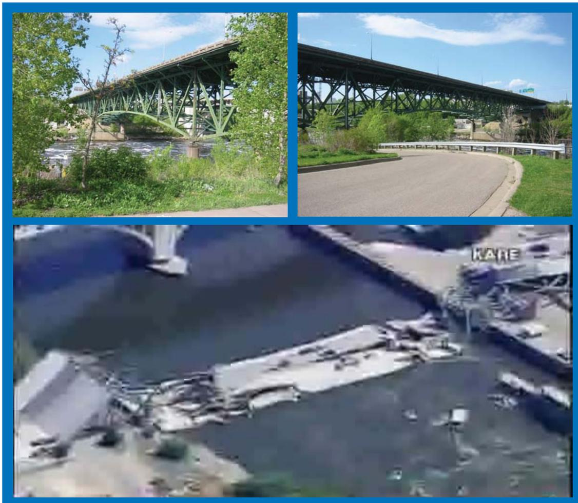
In the years prior to the collapse, several reports cited problems with the bridge structure. In 1990, the federal government gave the I-35W bridge a rating of "structurally deficient," citing significant corrosion in its bearings. Maintenance work was taking place in the weeks prior to the collapse included joint work and replacing lighting, concrete and guard rails. At the time of the collapse, four of the eight lanes were closed for resurfacing.
